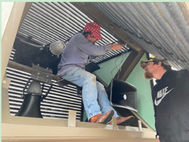
Campbellville workers installing the Speakers on the Tower.
